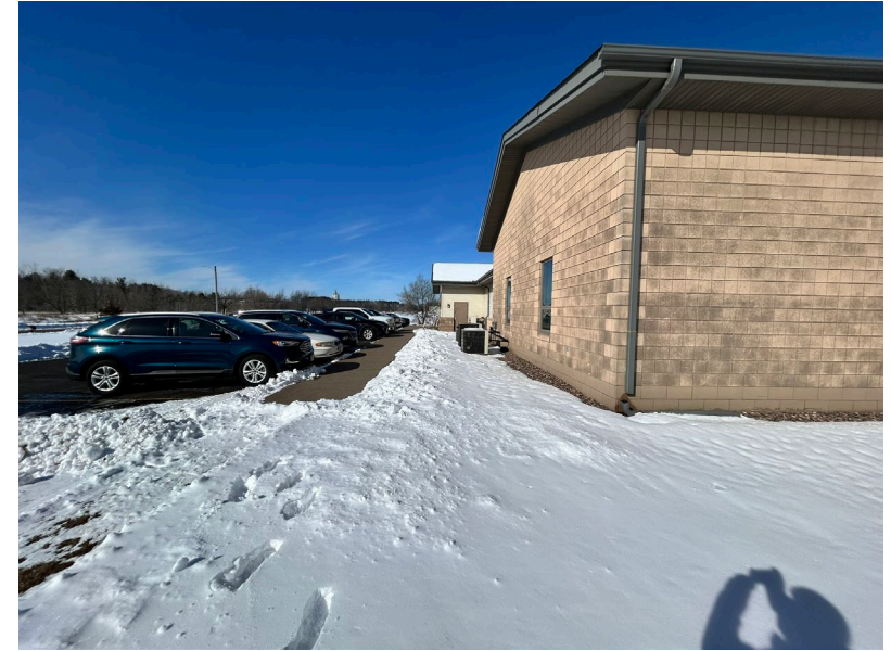
Southeast corner of the existing building, looking west.
