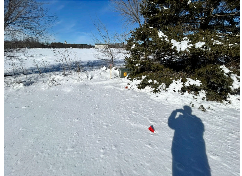
The second transformer on the west side of the existing building.
