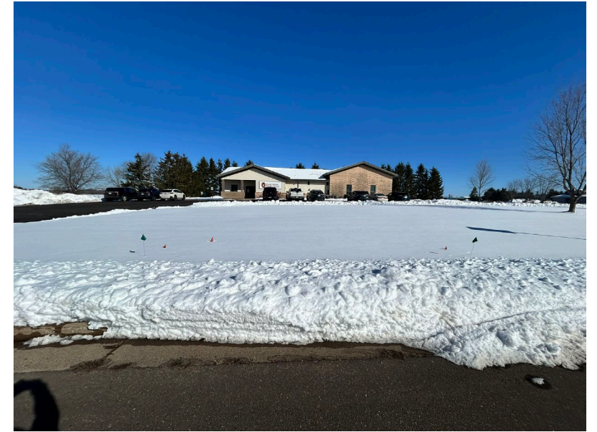
A view of the existing building, looking north.
