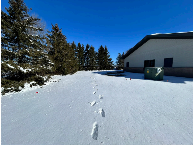
Southwest corner of the existing building, looking north.
