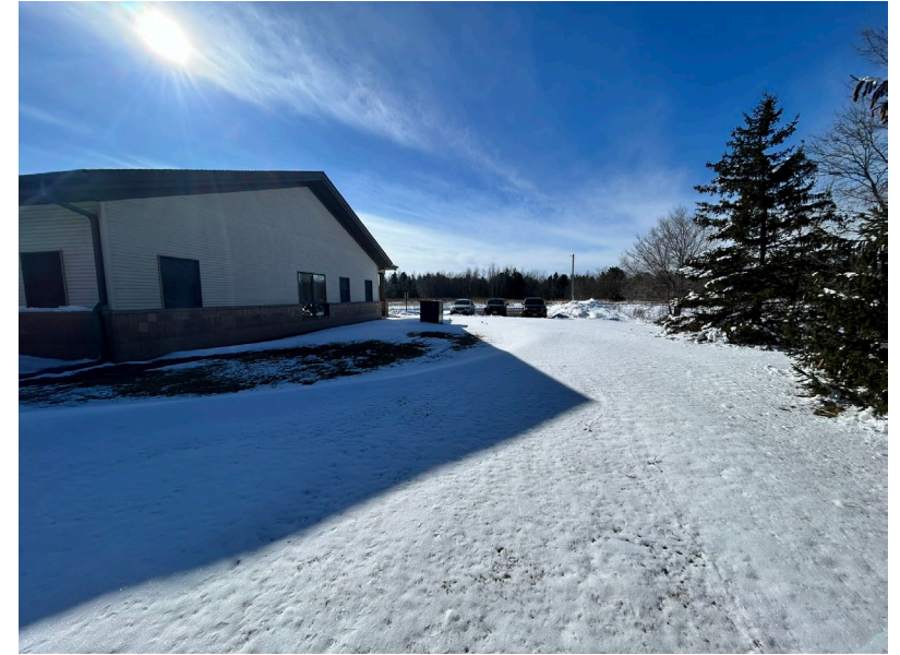
Northwest corner of the existing building, looking south.
