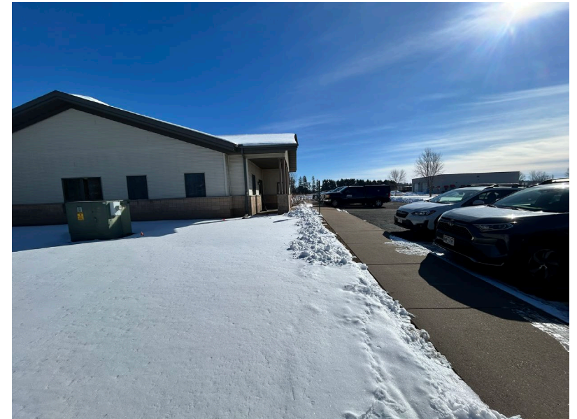
Southwest corner of the existing building, looking east.
