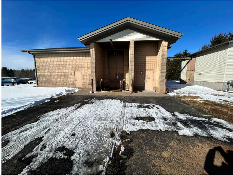
East side of the existing building, looking west.
