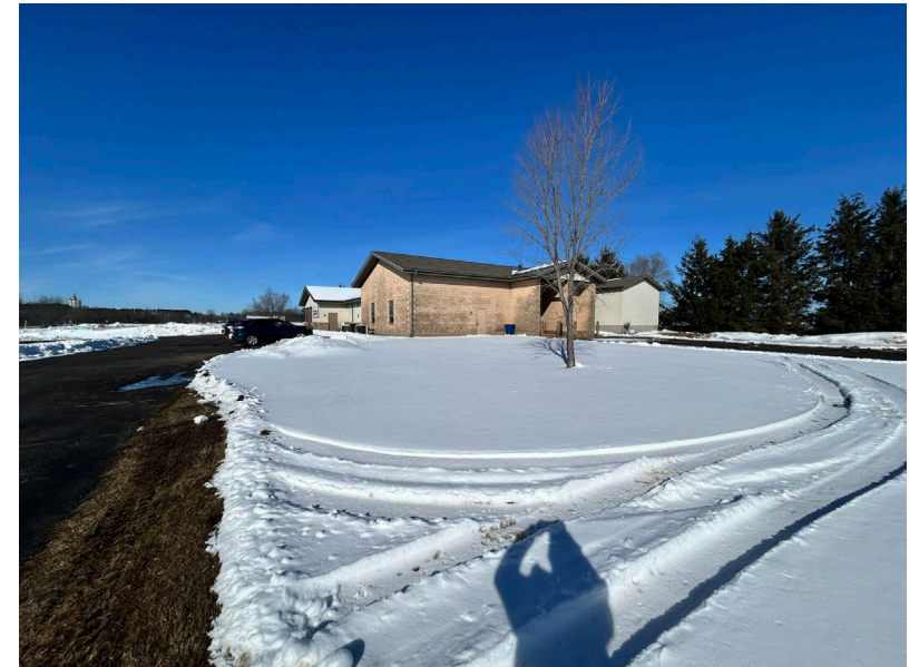
The existing landscaping on the southeast corner of the existing building.
