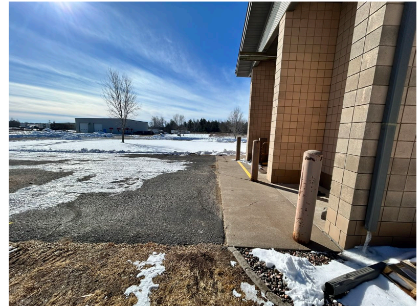
Northeast corner of the existing building, looking south.
