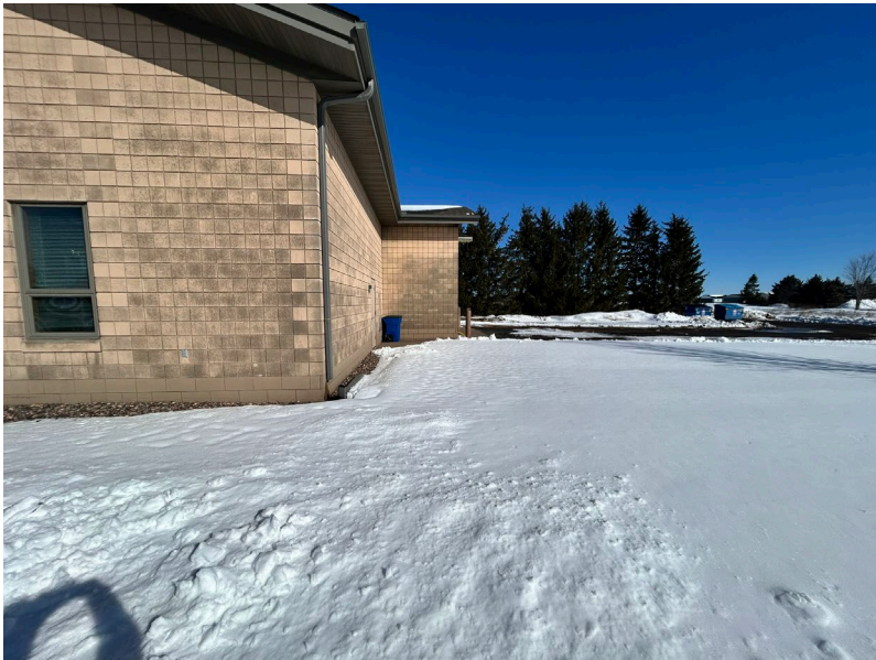
Southeast corner of the existing building, looking north.
