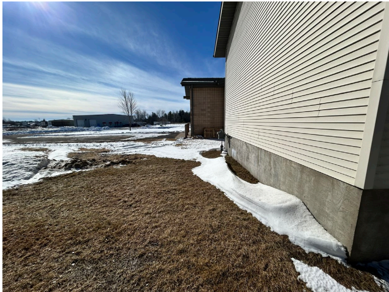
Northeast corner of the existing storage shed on site, looking south.
