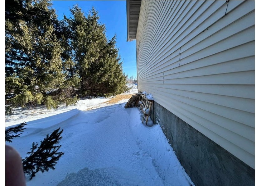
Northwest corner of the existing storage shed on site, looking east.
