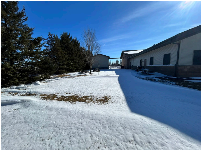
Northwest corner of the existing building, looking east.
