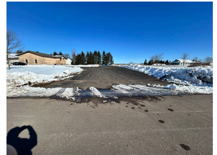
East driveway entrance, looking north.
