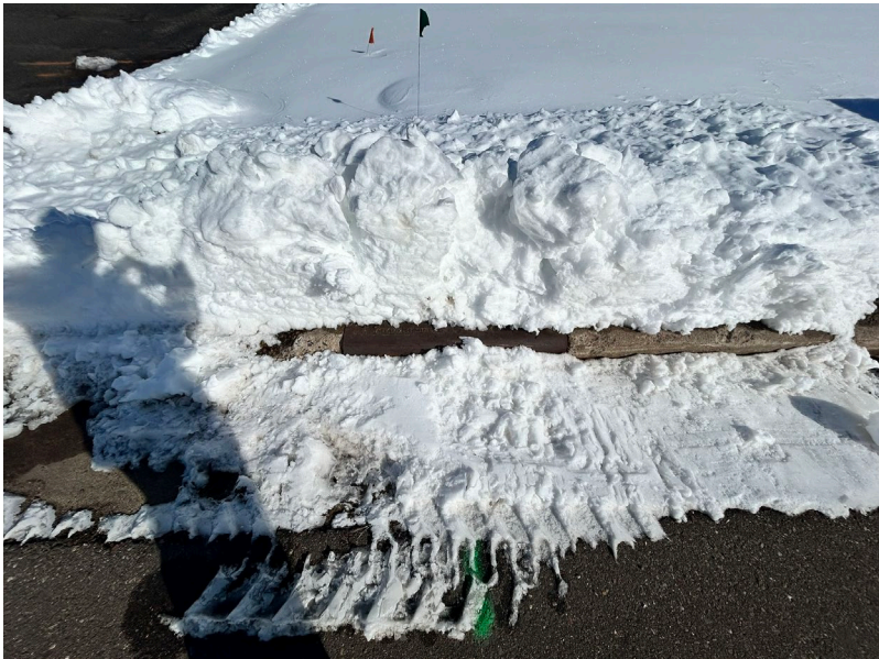
The storm sewer near the southeast corner of the west driveway..
