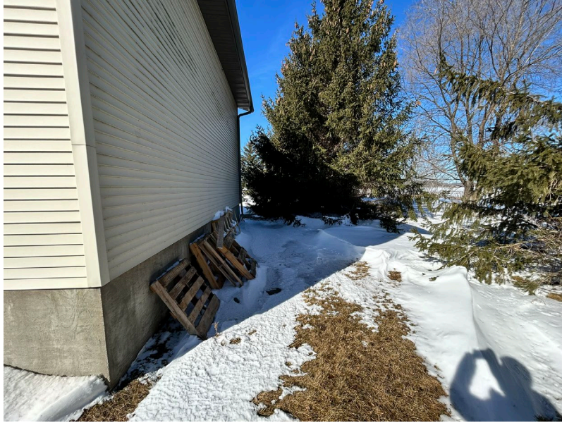
Northeast corner of the existing storage shed on site, looking west.
