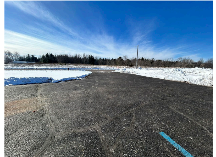
Looking south from west driveway.
